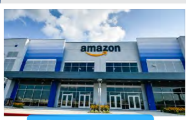
amazon DISTRIBUTION CENTER
